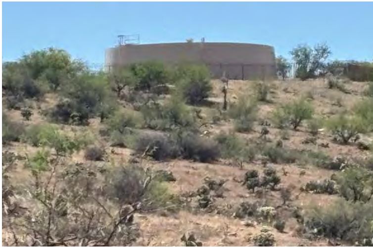
The 300,000 water storage tank
